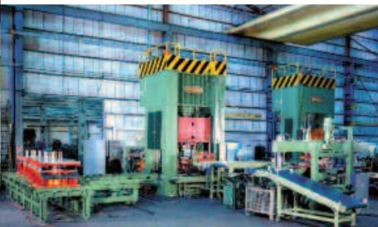
PRODUCTION LINE OF BOILERS
